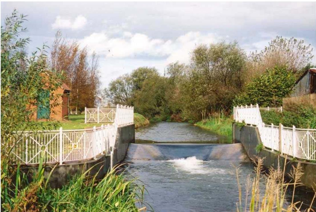
*A modern discharge monitoring weir of the flat-vee type. This type of weir is often favoured for its accuracy of flow measurement and suitability for both low and high flows. It is one of the best weirs for sediment conveyance, but tends to make fish migration difficult. Note that it is possible to create an attractive gauging weir that sits well in its surroundings.*
