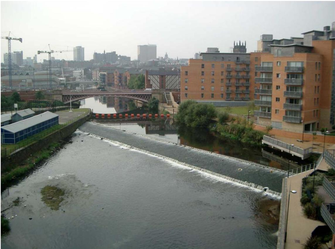
*Crown Point weir on the River Aire in Leeds is located in an area of renewal and development. The weir is diagonal to the flow to maximise the crest length and thereby reduce water level variation upstream. Note the new riverside walk on the right of the picture, and the historic bridge in the background (photograph courtesy of British Waterways).*
