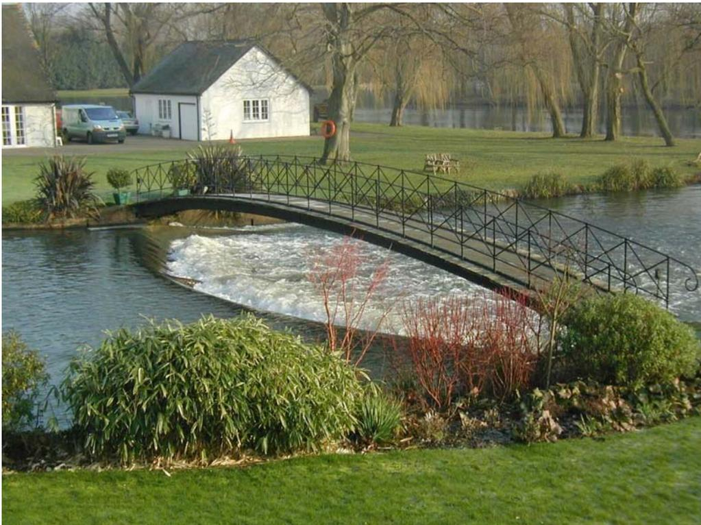
*Not all weirs can be designed to enhance the visual environment as much as this graceful structure with its arching form and matching elegant footbridge, but even a little extra thought at the planning and design stages can yield significant environmental benefits. Note that this weir has two fish passes, one on either flank.*
