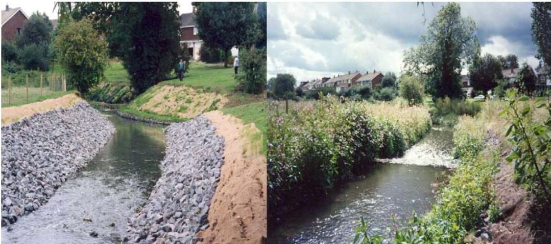
*The creation of a riffle in a small urban brook can look quite stark immediately after construction, despite the use of natural materials (rock). However, as the second photograph (taken one year later) shows, such works soon blend into the environment.*
