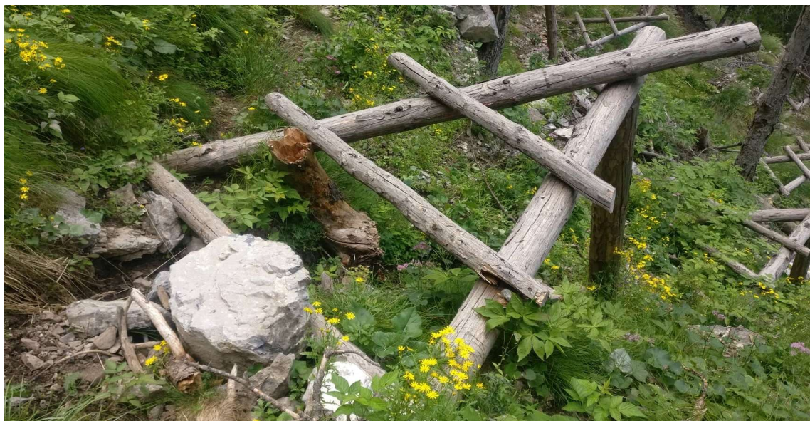
Figure 29. Wooden technical measures that reduces propagation probability of rockfall (Photo: Barbara Žabota, 2019).
