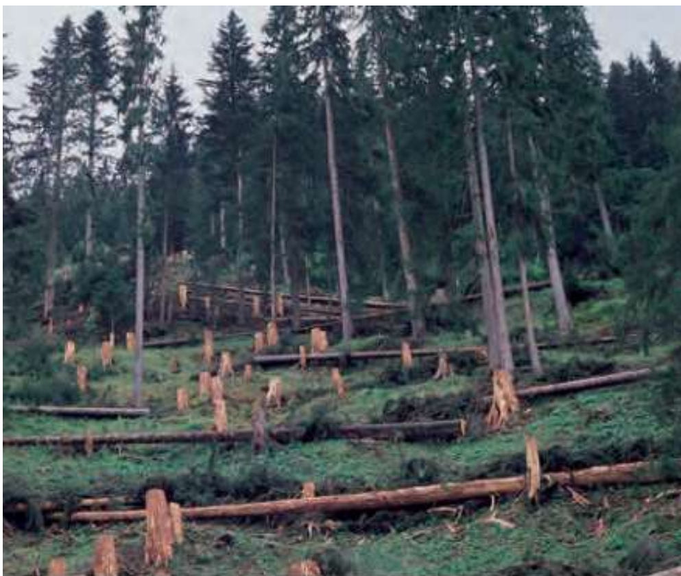
Figure 14. Rockfall protection by obstacles consisting of logs positioned on the slope (Photo: Bernhard Maier) (Dorren et al., 2007).
